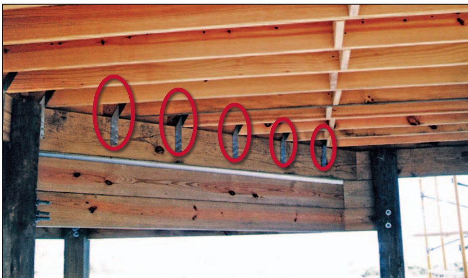
Figure 13-19. Proper use of metal twist strap ties (circled); solid blocking between floor joists
