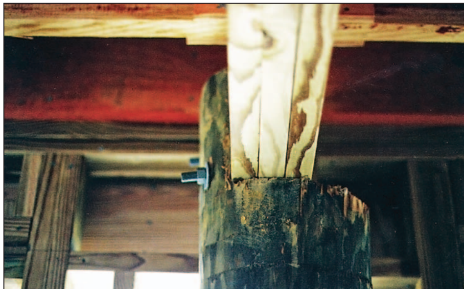
Figure 13-3. Improper overnotched wood pile
