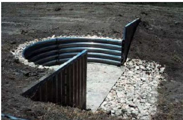
Figure TS14P-29 Grade stabilization structure
