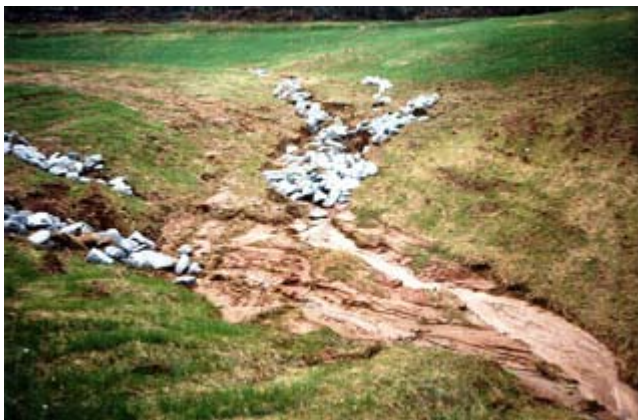
Figure TS14P-33 Rock placed in gullies arms the flow path on steeper slopes to prevent gully advance
