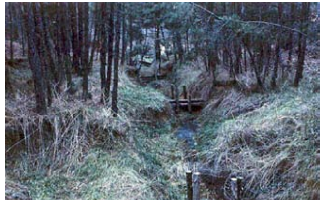
Figure TS14P-17 Early efforts to stabilize gully enlargement in the SC Piedmont used log check dams
