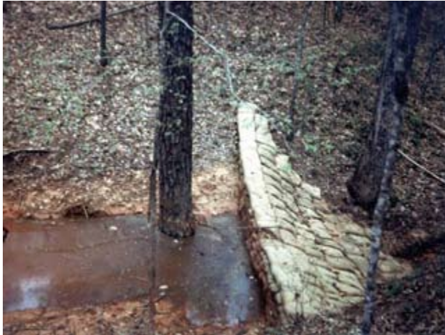
Figure TS14P-27 Soilcrete used to construct a small grade control structure
