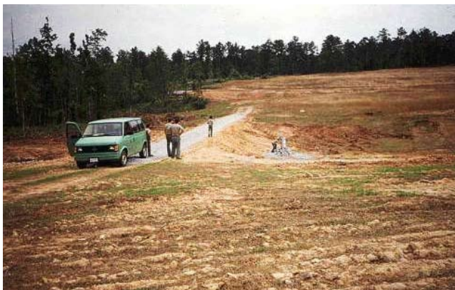
Figure TS14P-16 Active gully area reshaped with the flow from terraces going into a waterway, rather than adjacent gully areas
