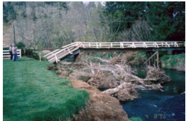
Figure TS14Q-2 Flood-damaged bridge in EWP program (Photo courtesy of Ben Doerge)
