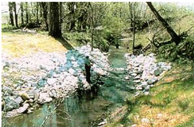
Figure TS14G-22 Grade control structure 1 month and 18 months after construction (Blue Creek, IL)
