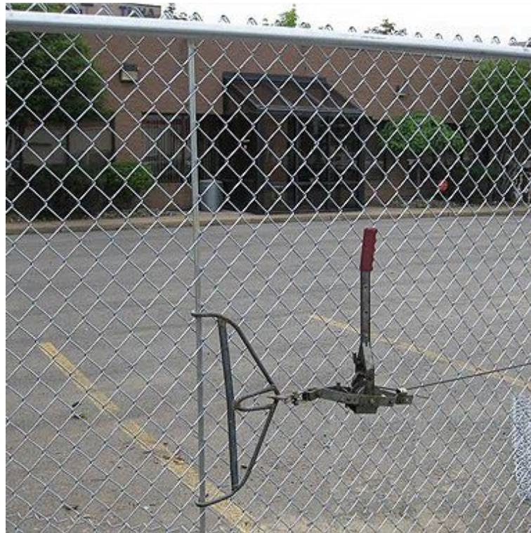
Figure 4-11 — Stretching fabric.
