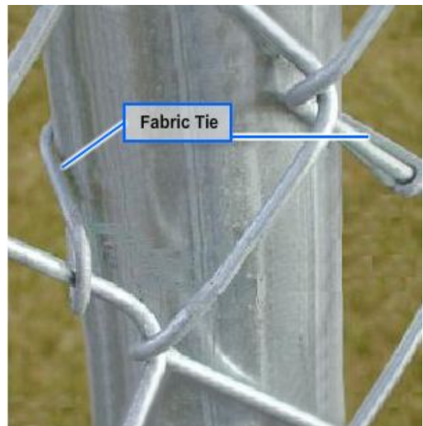
Figure 4-12 — Line post fabric tie.
