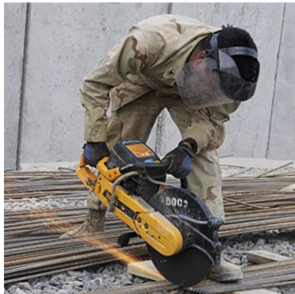
Figure 3-13 — Hand-held chop saw.
