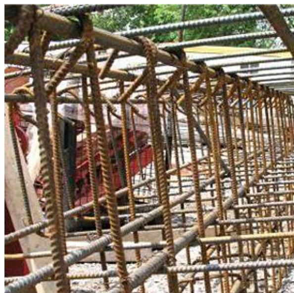
Figure 3-7 — Column ties.
