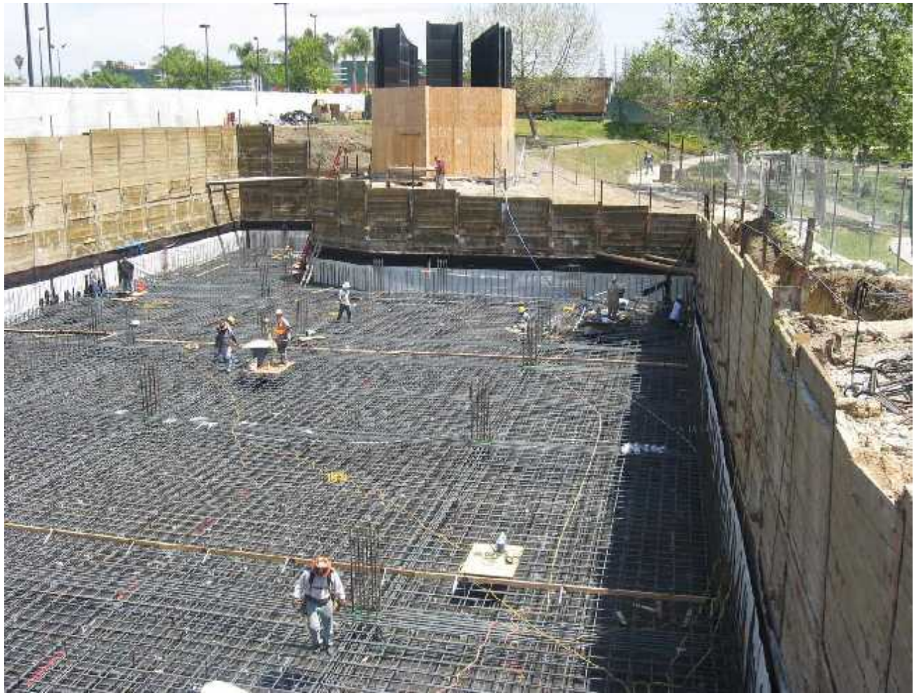
Figure 3-29 — Large floor slab.
