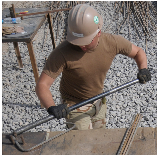
Figure 3-9 — Manual bending.
