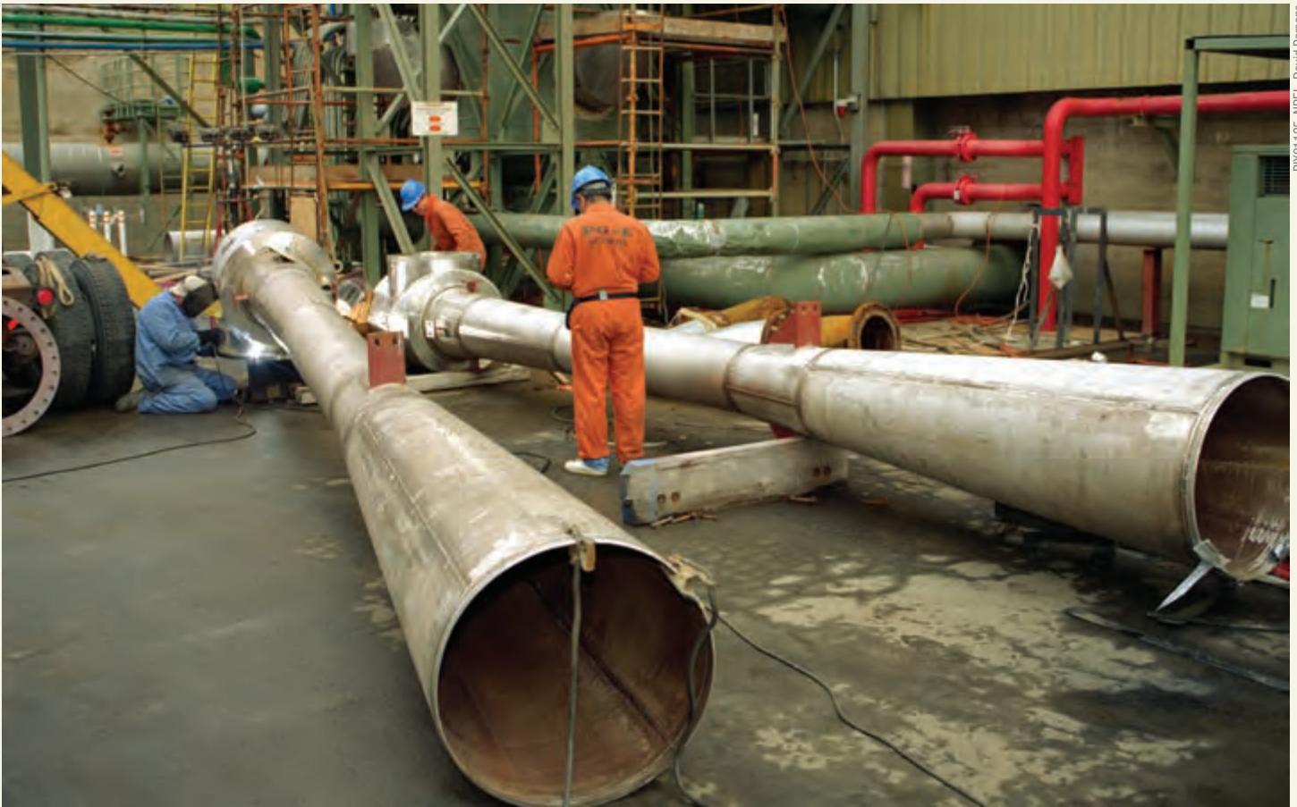
Workers install new piping at one of the geothermal power plants at The Geysers in northern California.
