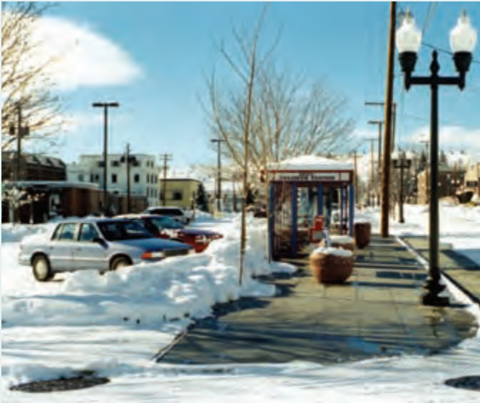
In Klamath Falls, Oregon, the city applies direct-use geothermal for keeping sidewalks and bridges clear and dry after a snowfall.
