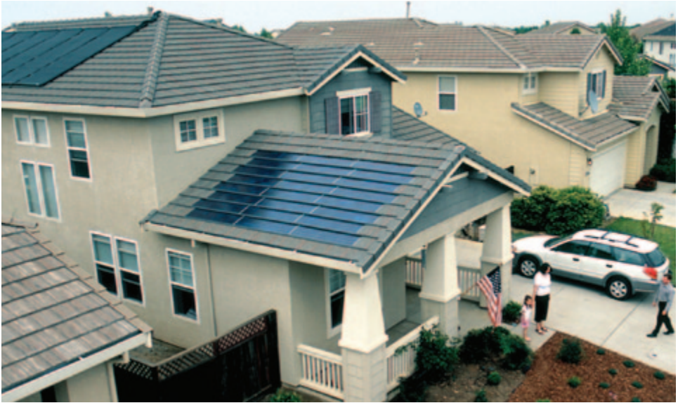
This solar home in Davis, California, uses EnergyTiles ® made by BP Solar.
