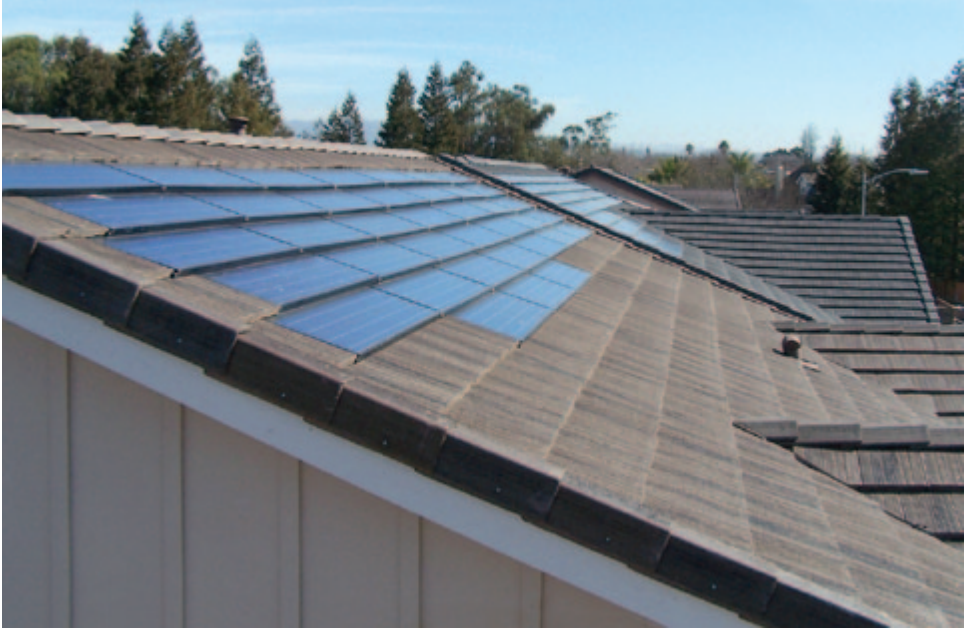
A roof-integrated solar electric system on a home in San Jose, California.
