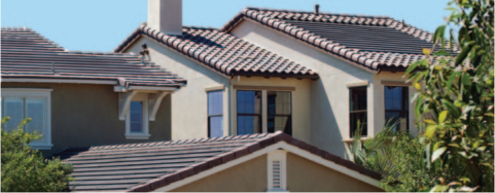
Solar homes in California with SunPower Suntiles® integrated into their roofs.
