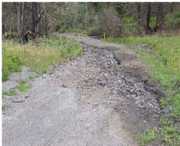
Figure 7-16 — Example of an uncrowned traveled way.
