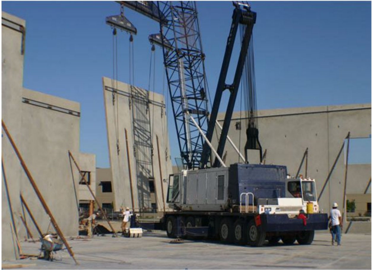
Figure 3-20 – Precast panels being erected by use of crane and spreader bars.
