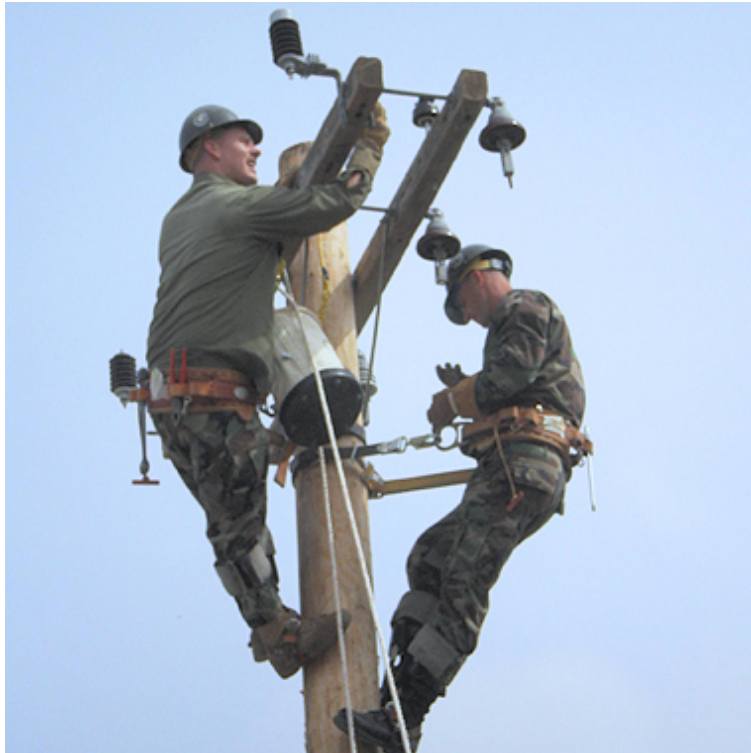
Figure 4-1 – Construction Electricians performing pole climbing evolution.
