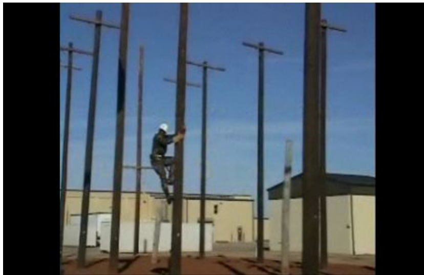
Figure 4-12 – Ascending utility pole.
