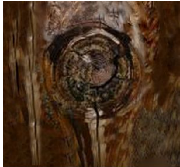
Figure 4 - 11 – Examples of inspectable items.
