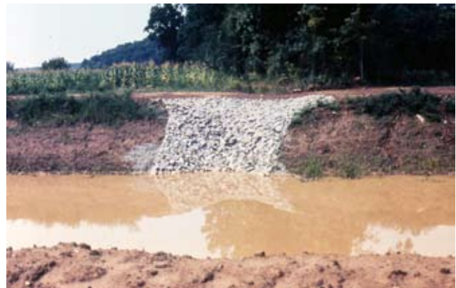
Figure TS14C-4 Toe of the slope lined with stone to control erosion
