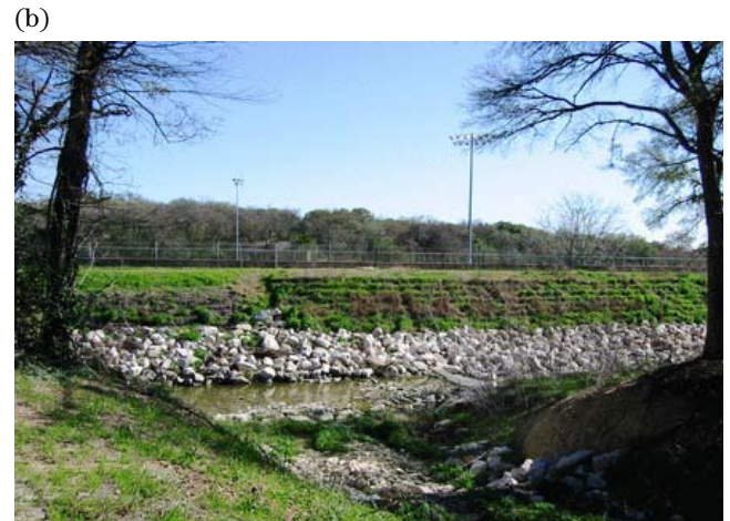
Figure TS14A-9 Before and after pictures of project, Shoal Creek in Austin, TX. The toe of the slope was protected with riprap and the bank shaped above the protected toe. (Photo courtesy of City of Austin, TX)
