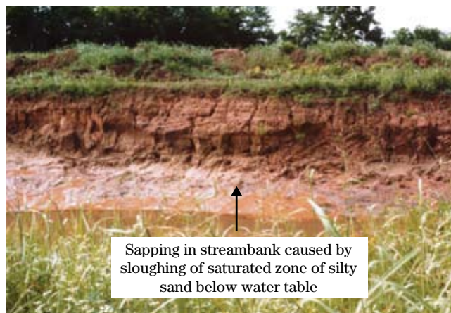
Figure TS14A-17 Sloughing of saturated low plasticity zone in lower streambanks caused by seepage forces
