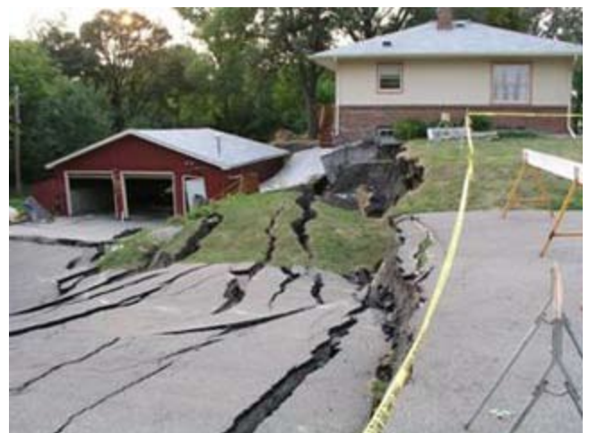
Figure TS14A-6 Typical slope stability failure in clay soil type. Failure is a low-radius, deep rotational failure. (Photo credit City of Fargo, ND)
