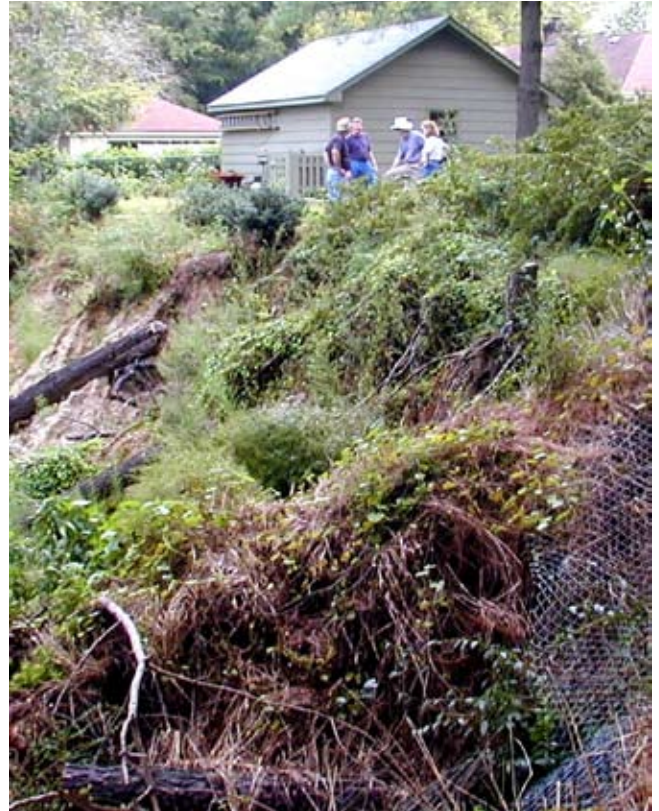
Figure TS14A-4 Failed streambank in Tarboro, NC, following high channel flows following Hurricane Floyd. Erosion of the toe caused bank instability in the slope. Measures to protect the toe of the slope are essential, in addition to assuring stability of the system.
