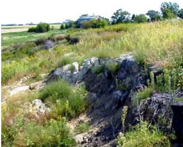
Figure TS14A-5 Shallow sloughing failure in zone of saturated sand
