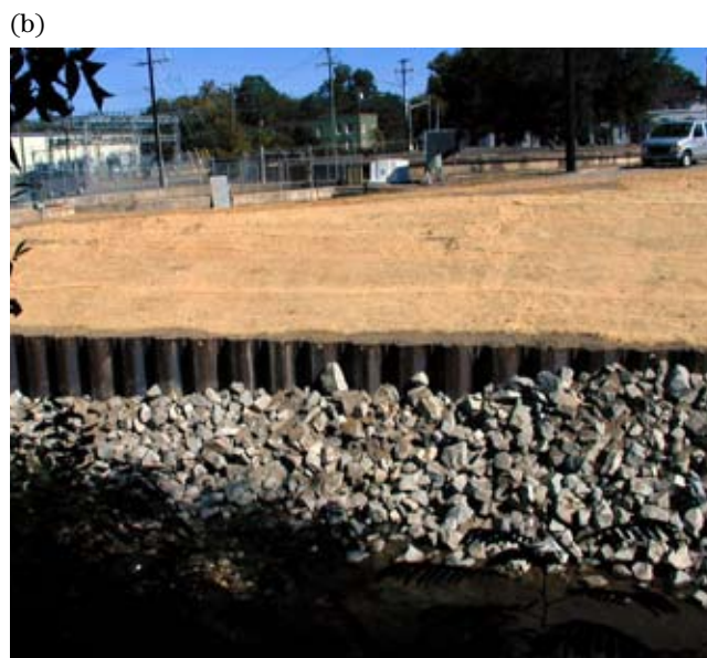
Figure TS14A-11 Sheet pile wall at toe of slope in Tarboro, NC. Vegetation will be established above wall. Note erosion control fabric.
