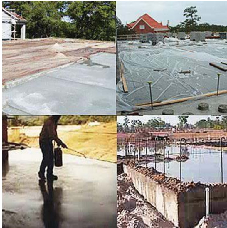
Figure 10-23 — Examples of alternative methods to retain moisture during initial hydration.
