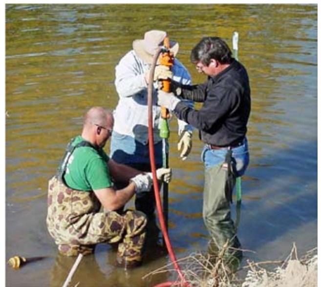
Figure TS14E-4 Driving soil anchor with a 30-lb jackhammer
