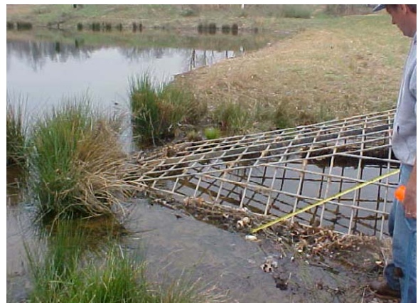
Figure 1.1: Abnormally high permanent pool – Water spills into 2- year weir because beavers have clogged the low flow orifice.
