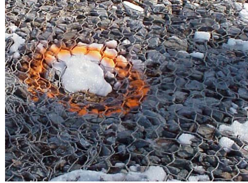
Figure 2.4: Marking a hole in gabion fabric
