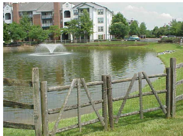
Figure M7.2: Surface aerator / fountain.
