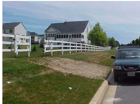
Figure 1.12: Pond with good access to public road.
