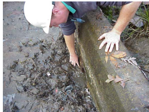
Figure M2.3: After clog is removed.
