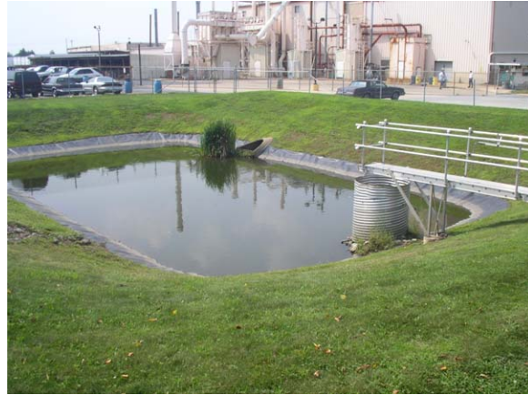
Figure 1.3: Riser without trash rack
