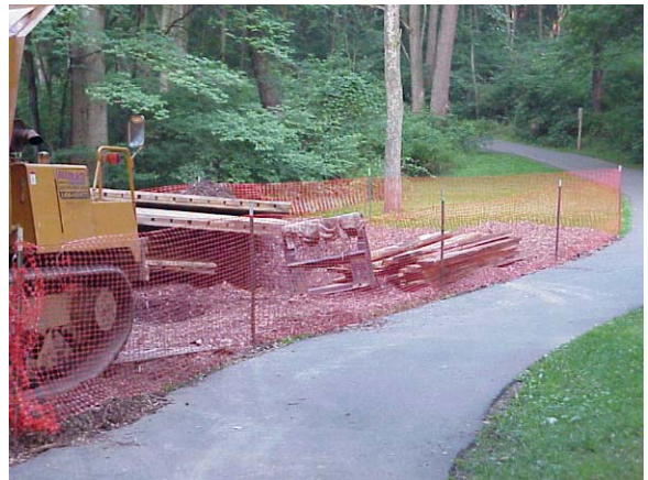
Figure M6.5: Paved access road.
