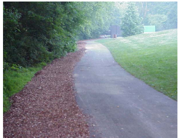
Figure 1.15: Temporary access road widening
