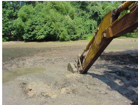
Figure M5.4: Mechanical dredging with backhoe.
