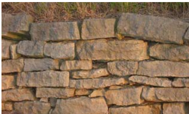
Figure TS14M-1 Dry stacked stone wall
