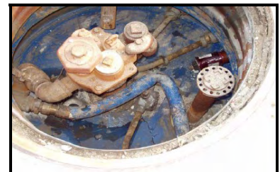
Flexible piping is kinked
