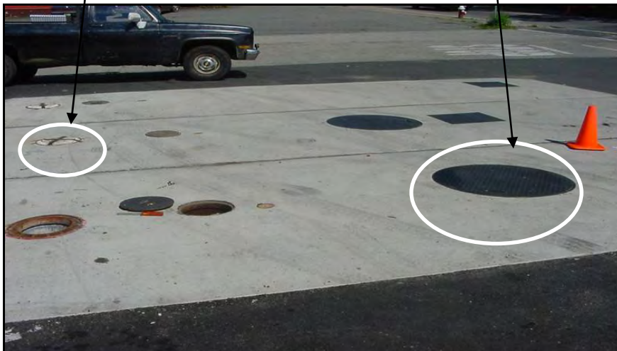
View of sump lids
