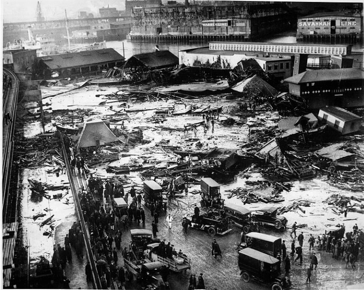
Figure 1. Aftermath of molasses tank failure
