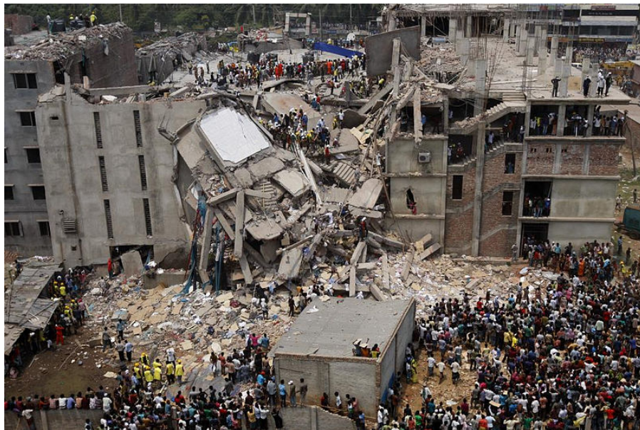
Figure 2. Aerial view of collapse.
