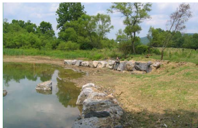
Figure TS14H-6 Rock vane
