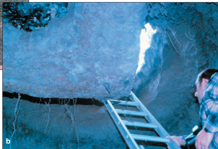
Figure 9 Pit subsidence under the corner of a house from (a) above and (b) below ground.
