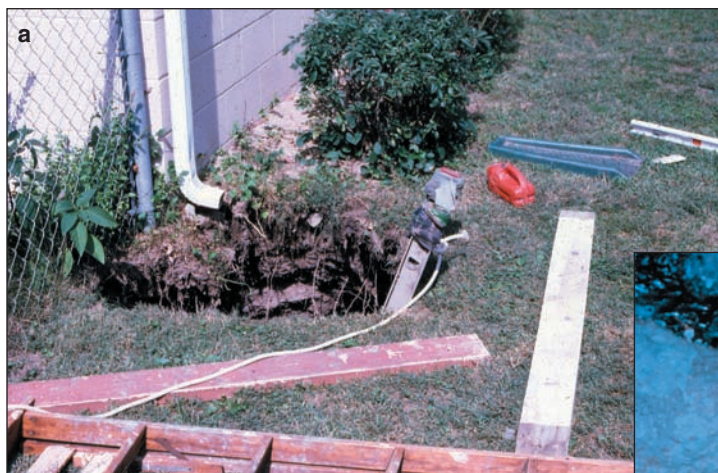
Figure 9 Pit subsidence under the corner of a house from (a) above and (b) below ground.
