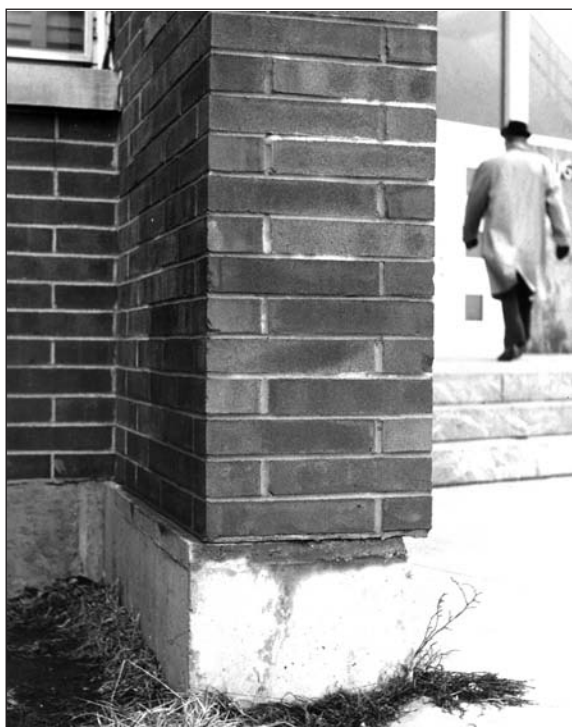
Figure 28 The largest movements are at the edges of the long continuous wall. At this point, the brick wall is being pushed off the foundation.
