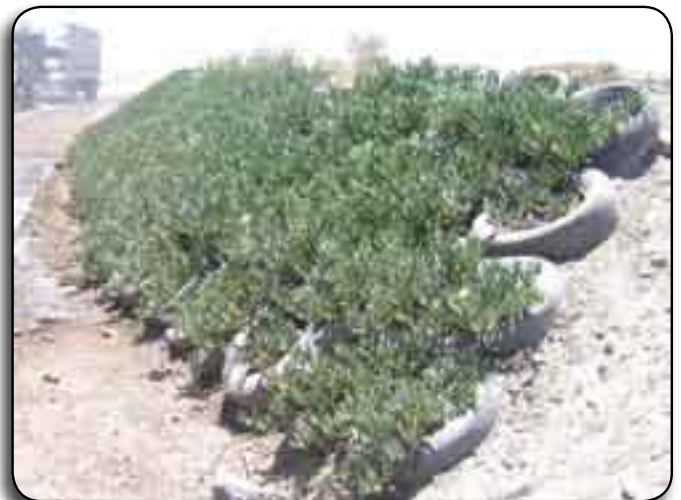
Whole tire erosion control wall, Los Arroyos, Mexico
