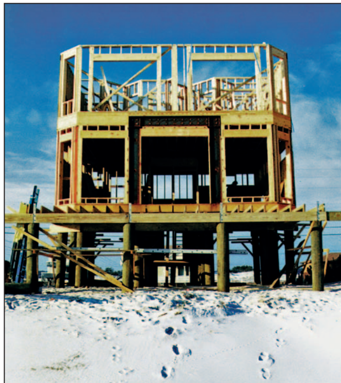
Figure 9-25. Steel moment frame with large opening
