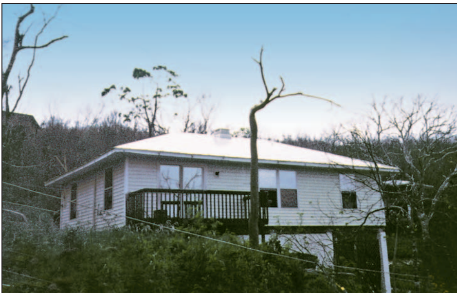
Figure 9-27. Hip roof that survived high winds with little to no damage, Hurricane Marilyn (U.S. Virgin Islands, 1995)
