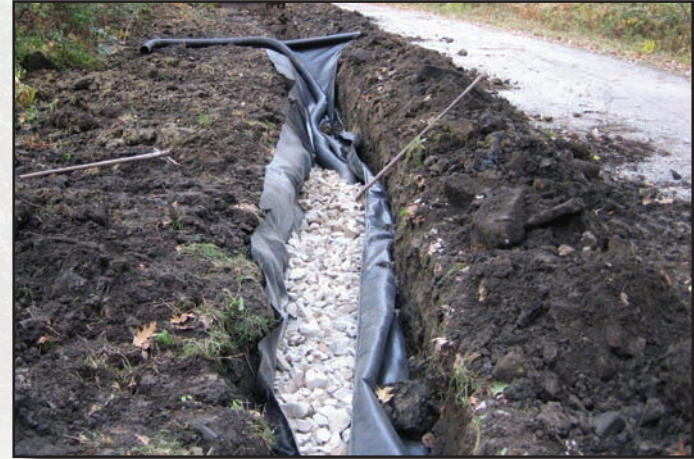
Figure 2.7—Free draining stone.
