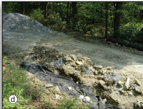
Figures 2.8a through 2.8d—French drain construction sequence.
