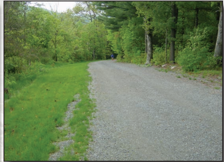
3.4b—Outsloped roads eliminates ditches.
