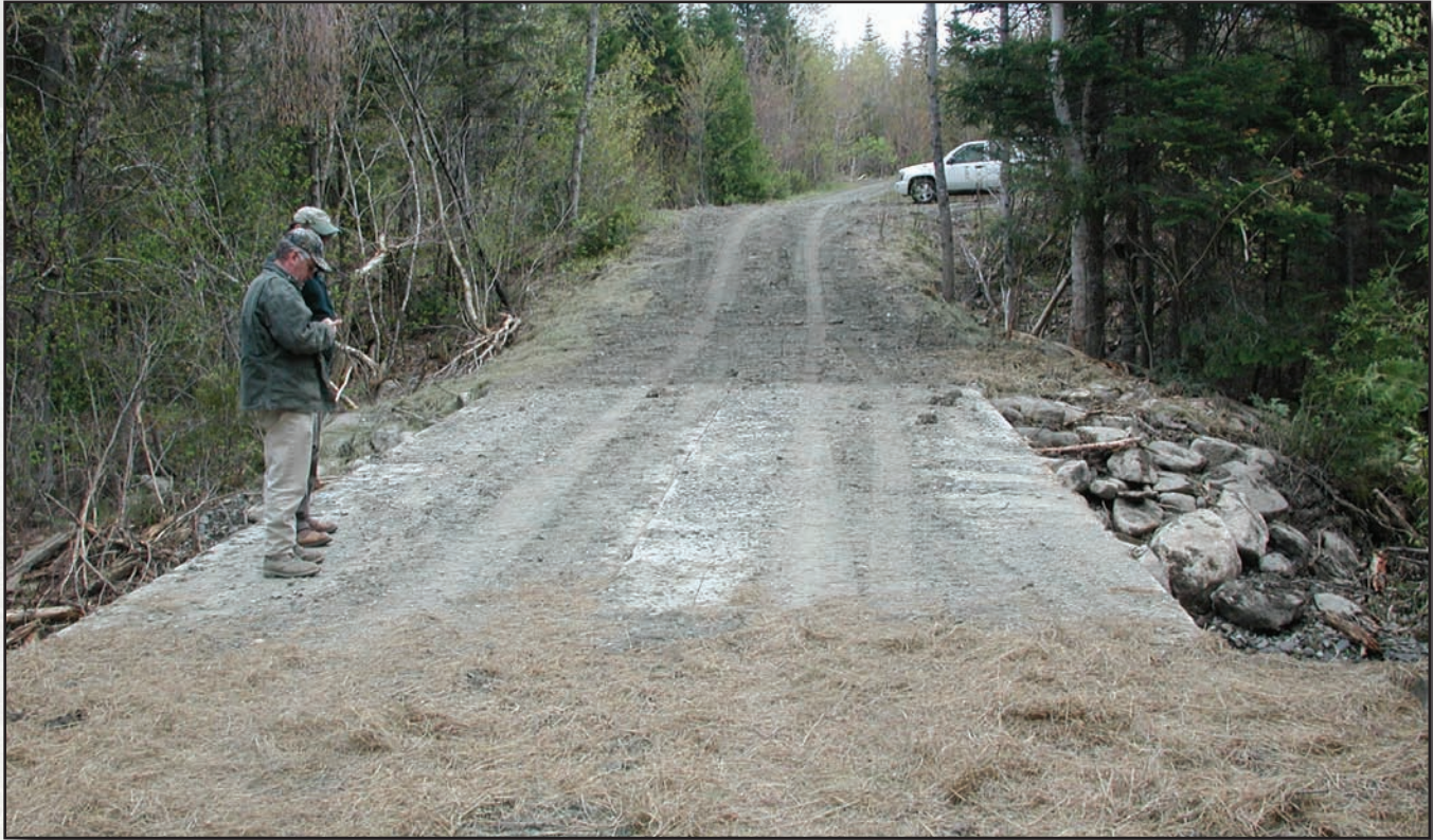
Figure 9.1—Road Assessment and monitoring.
