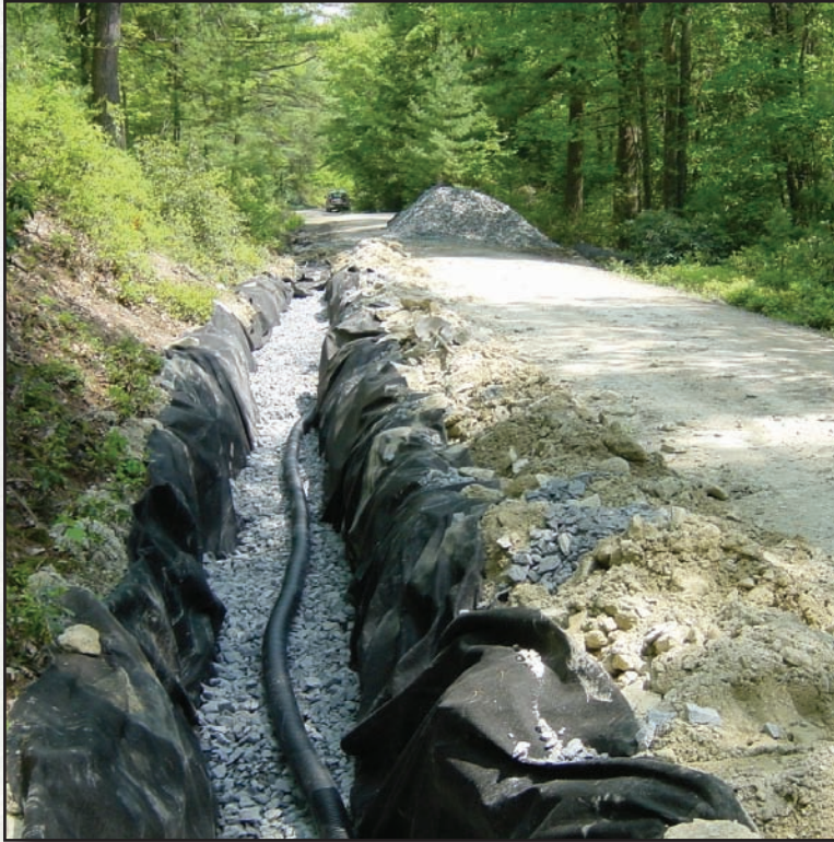
Figure 2.5—This drain collects water from springs and seeps under the road ditch.
