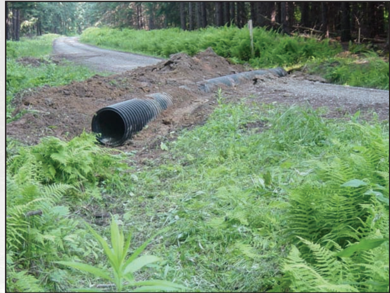
Figure 5.7—A shallow cross pipe being installed: The cross pipe shown is partially installed. Notice that the pipe outlet is at the elevation of the existing ground, no outlet trench or tail ditch is required. The top of the pipe is ABOVE the existing road surface. The required pipe cover is obtained by importing fill. When completed, the fill will create a grade break over the pipe.
