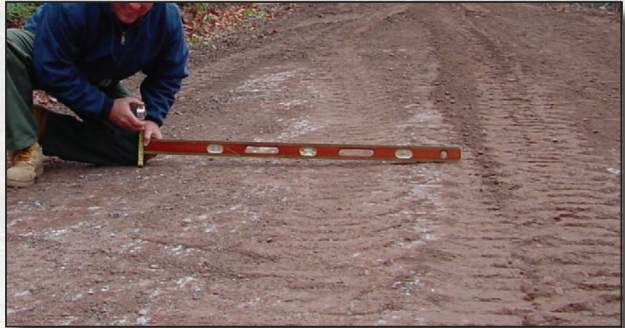
Figure 3.6—A road's sideslope can be measured using a level and tape measure. The road should drop 2 to 3 inches over the 4-foot length of the level used in the picture above.
