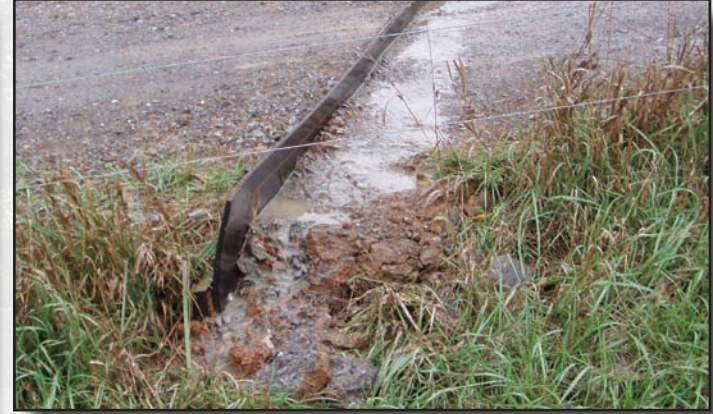
Figure 3.15—A completed diversion directs surface drainage off the roadway and into a field.
