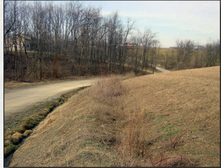
Figure 7.11—The interceptor swale pictured here catches the runoff from a large field before it enters the road.
