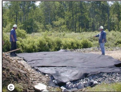
Figures 2.16a through 2.16d—French mattress construction sequence.
