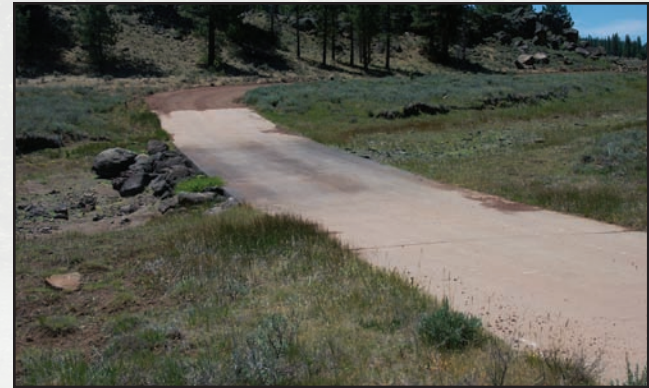
Figure 6.5—Concrete ford crossing.
