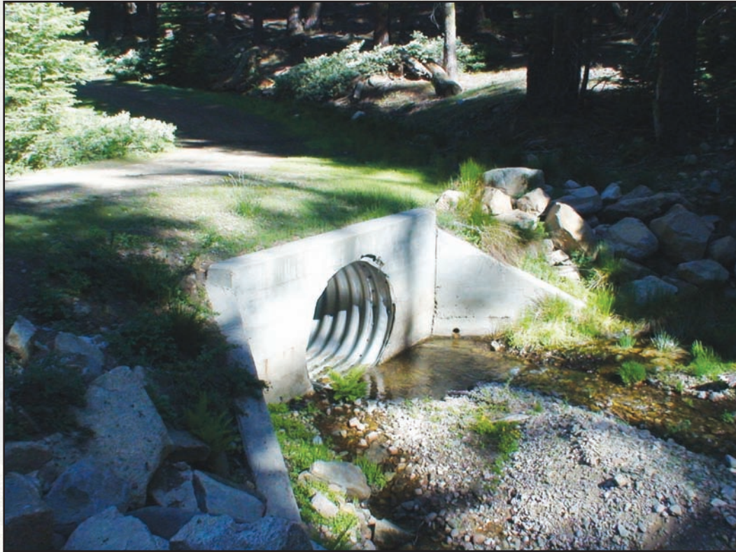
Figure 5.14—Headwall with wingwalls.
