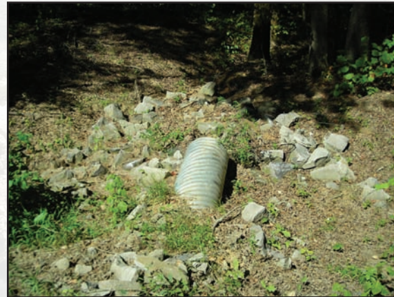
Figure 5.3—Culvert outlet is well armoured.
