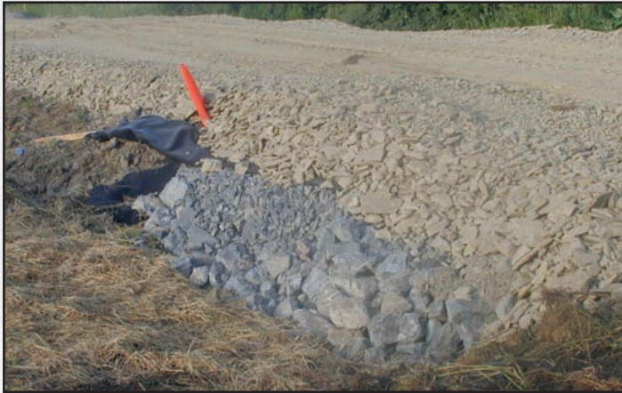
Figure 2.11—Side view of a large French mattress.
