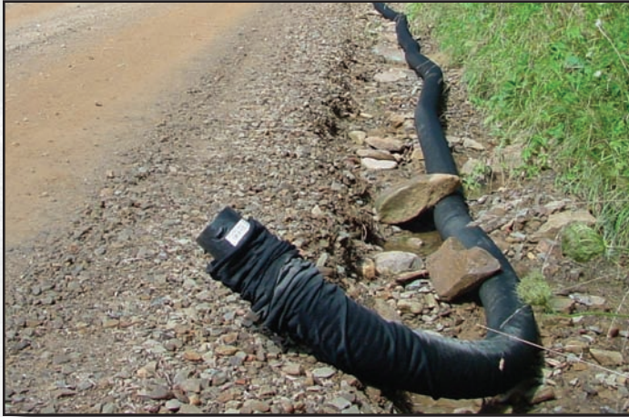
Figure 2.6—Perforated plastic pipe.
