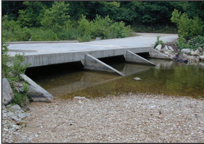
Figure 6.7—Vented ford or low-water bridge.
