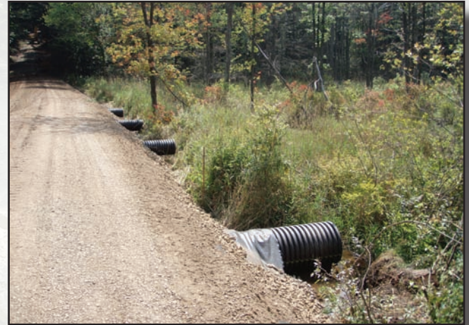
Figure 2.19—Permeable fill with culverts spreads surface flows.
