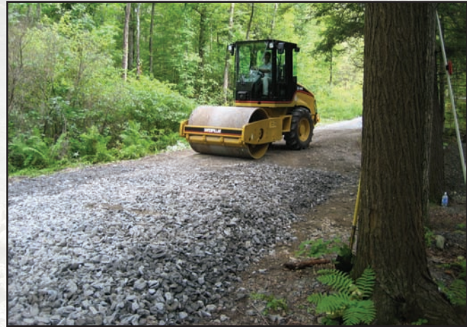
Figure 2.25—Roller compacts each of lift aggregate.
