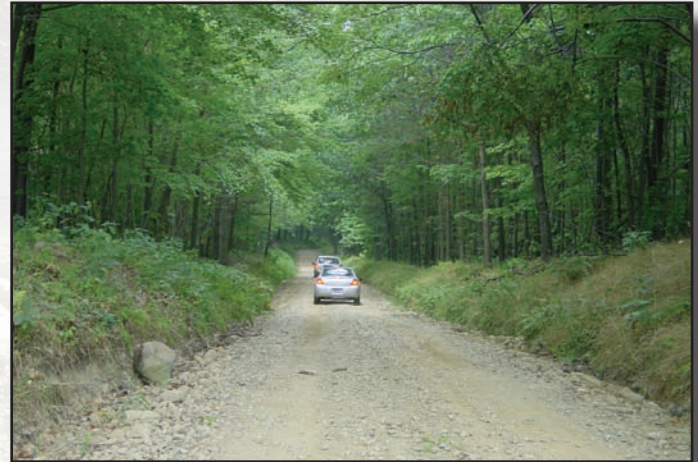
Figure 4.7—Example of an entrenched roadway.
