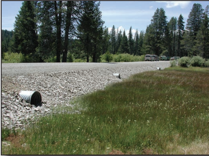
Figure 2.20—Permeable fill with culverts.
