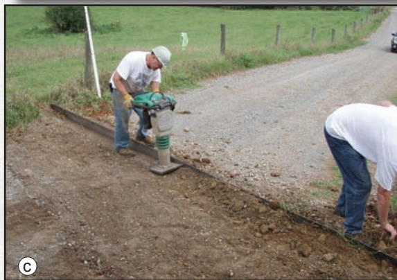
Figures 3.18a through 3.18d—Belt diversion construction sequence.
