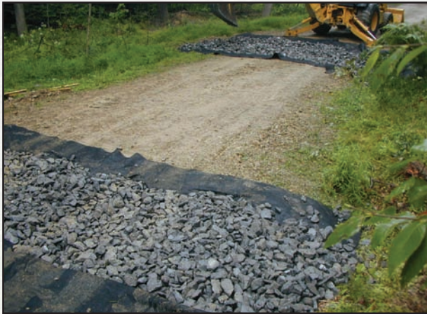
Figure 2.15a—Small mattresses installed to drain several springs and seeps.
