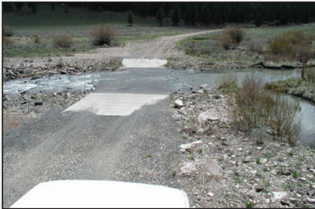
Figure 6.6— Low-water crossing.
