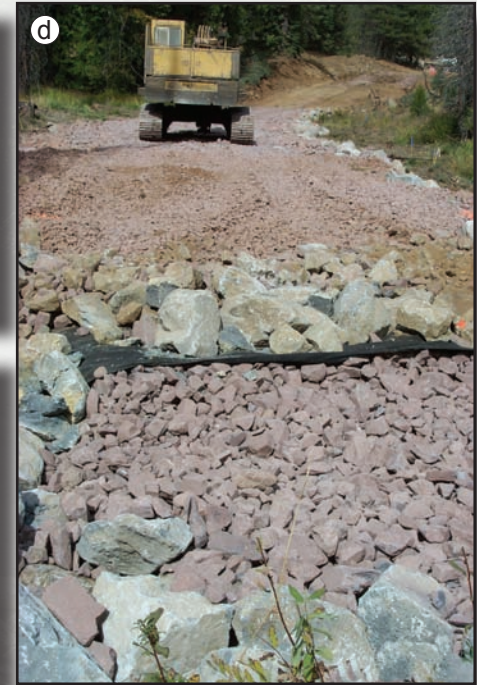
Figures 2.22a through 2.22d—Permeable fill construction sequence.
