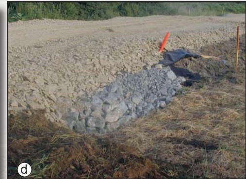
Figures 2.16a through 2.16d—French mattress construction sequence.
