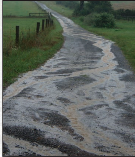
Figure 3.12—Low-volume access roads, such as the one pictured here, are ideal candidates for diversions.
