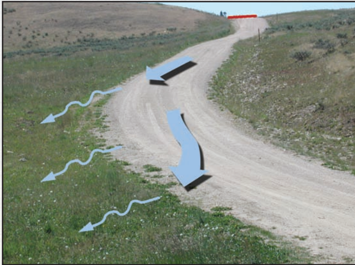
Figure 3.4a—Outsloped road disperses flow.
