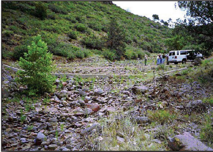
Figure 6.10—Jersey barrier in Arizona provides safe, low maintenance access to forest roads.
