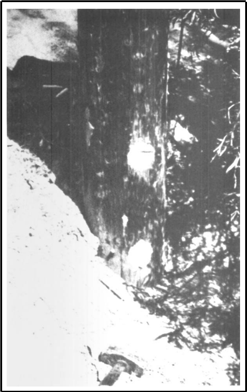
Figure 6 Pole Restoration Using Epoxy Resins, Fibers and Fillers
