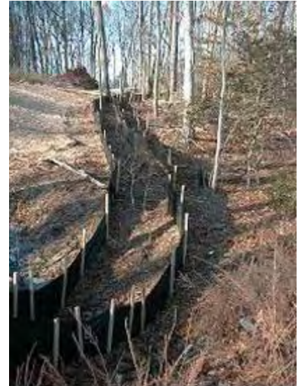
Silt fences prevent the offsite transport of sediment
