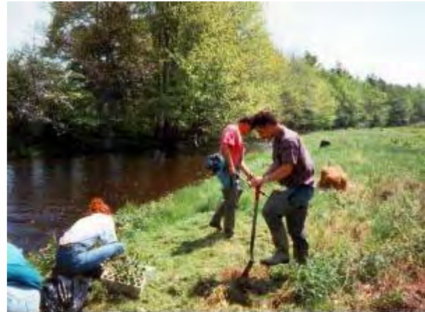
Buffers at the perimeters of construction sites are similar to agricultural buffers in that they trap sediments and remove pollutants in runoff from exposed areas (Source: Nova Scotia Department of Agriculture and Fisheries, 2000)
