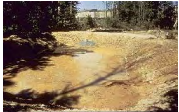
Sediment basins are used to trap sediments and temporarily detain runoff on larger construction sites
