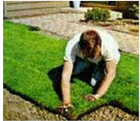
Grass sod is laid on exposed soil to stabilize the soil and to reduce the velocity of storm water runoff (Source: Landscape USA, no date)
