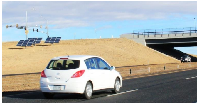
Figure 4. Solar Array on E-470
