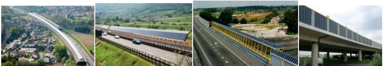
Figure 1. PV Arrays in Noise Barrier
