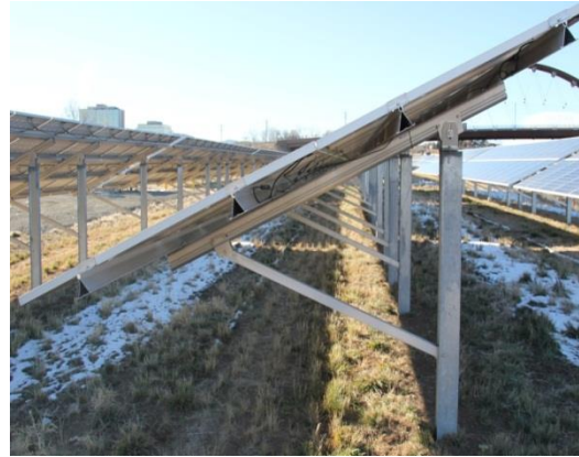
Figure 9. DFC Support Structure Example
