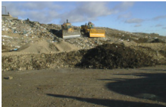
Figure 6.2: Bulldozers working in a landfill.
