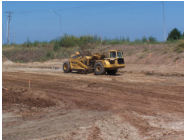
Figure 5.2: An example of construction machinery.
