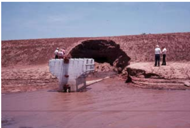
Figure 45-1 Failed embankments
