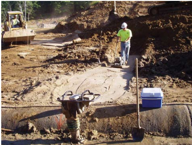
(e) Filter diaphragm being constructed to side of principal spillway conduit
