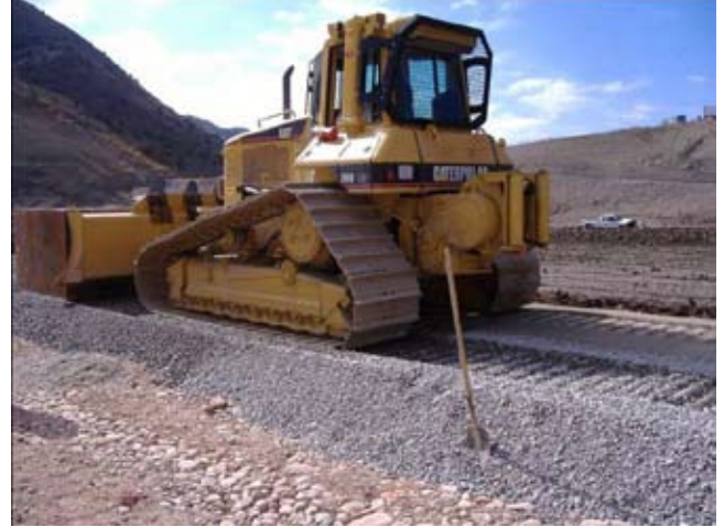
(f) Filters are then uniformly spread and compacted according to specifications.
