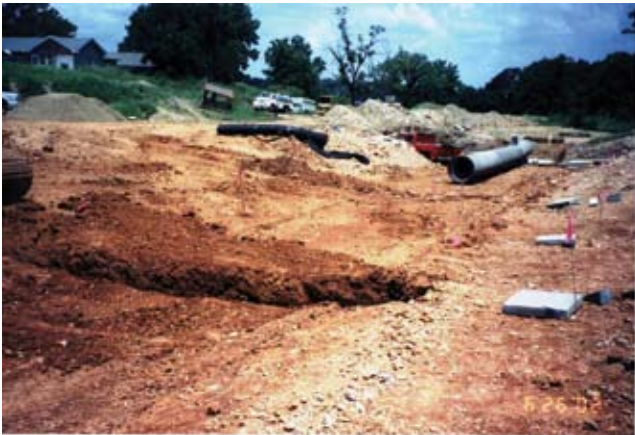
(a) Principal spillway excavated to grade prior to excavating filter diaphragm
