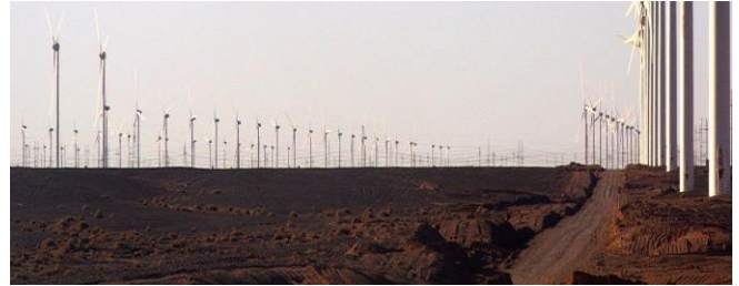
Wind farm in the Gansu province of China
