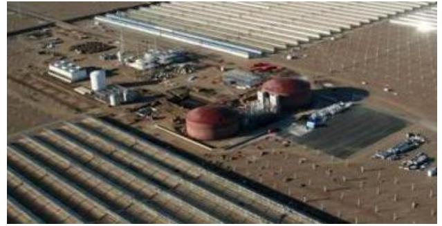
Two-Tank Indirect TES at Andasol1 in Spain Image source: greenthoughts.us
