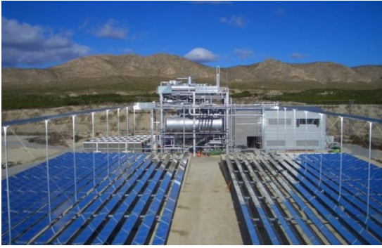
Multiple Absorbers in a CLFR system
