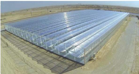
Enclosed Parabolic Trough CSP Facility Image Source: Greentechmedia.com
