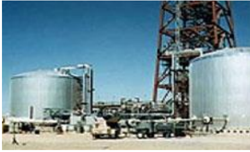
Two Tank Direct Molten Salt TES at the Solar Two Power Tower Plant Image source: NREL
