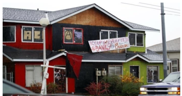
Vacant and Abandoned House
