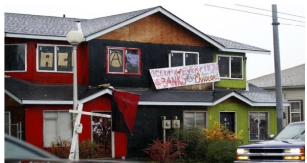
Vacant and Abandoned House
