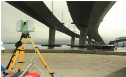
3D scan survey of the west span of the San Francisco-Oakland Bay Bridge
