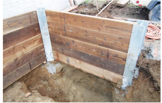
Steel Pilings used with Wood Beams
