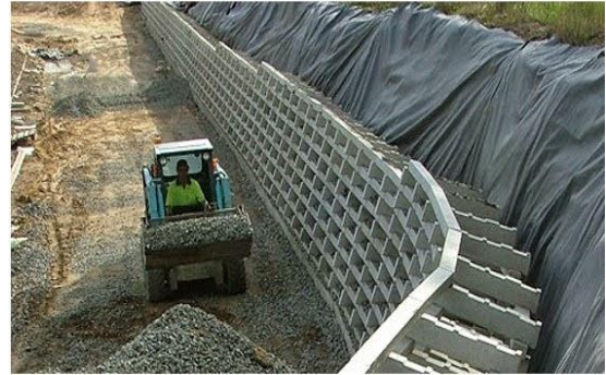
Timber and Concrete Crib Walls
