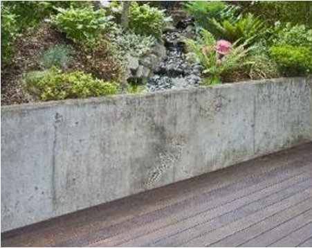
Steel Reinforced Concrete Wall
