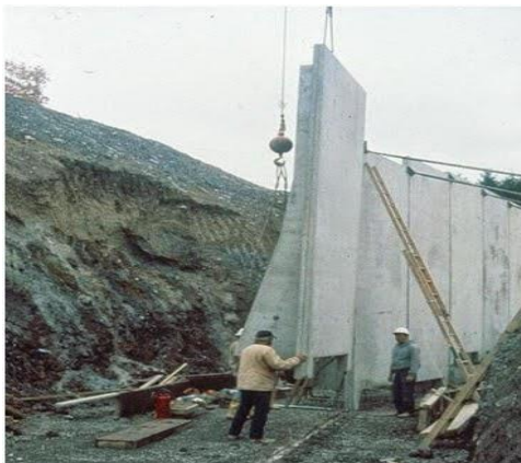
Pre-Cast Concrete Counterfort Retaining Wall
