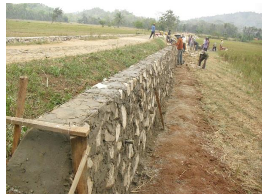
Wall made from Mortared Field Stones
