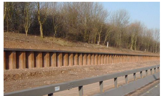
Sheet Piling Retaining Walls
