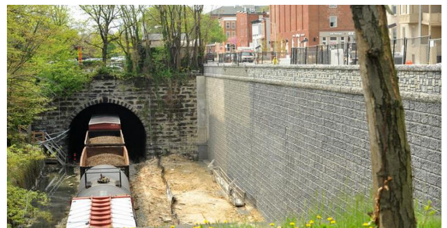
New Retaining Wall at East 26 th Street Image source: Baltimore Sun
