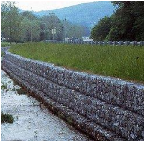
Gabion Wall along a Roadside Stream
