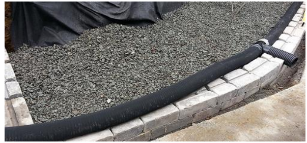
Sock Pipe Drainage
