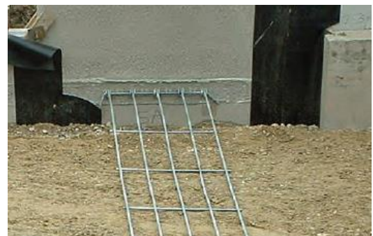
Bar Mat Soil Reinforcement Image Source: reinforcedearth.com
