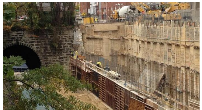
Rebuilding of the Wall Following the Collapse Image source: Baltimore Sun
