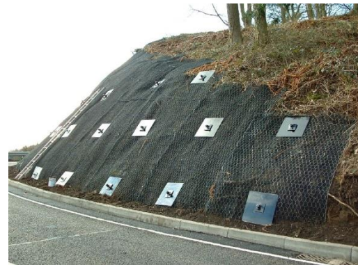
Soil Nailed Slope Support System (attached to wire meshing)
