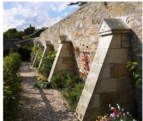
Culross Palace Gardens - Buttress Wall
