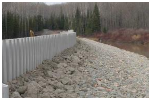
Vinyl Sheet Piling Wall
