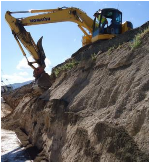
Heavy Equipment (imposing a surcharge load on the excavated slope below)
