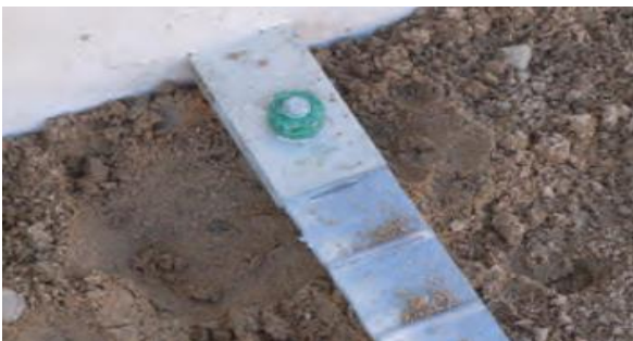
Tie Strap Soil Reinforcement Image Source: reinforcedearth.com
