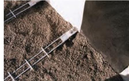
HA Ladder Soil Reinforcement Image Source: reinforcedearth.com
