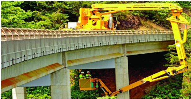
Bridge Inspections Team Image Source: Oregon DOT
