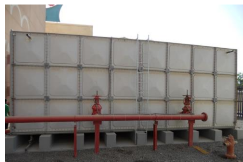
Prefabricated Sectional Water Tank Image Source: ParkitThere.com
