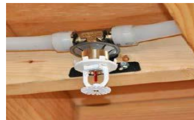
Residential Sprinkler with PEX Piping and Fittings
