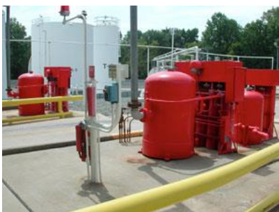
Dry Chemical Fire Extinguishing System Image Source: iafire.com
