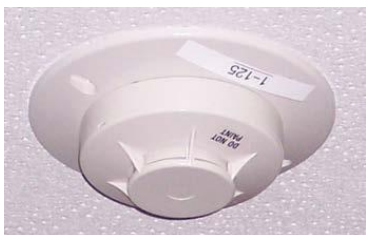
Spot Type Smoke Detector
