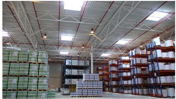
Warehouse with an ESFR system Installed Image Source: realestateinspain.wordpress.org
