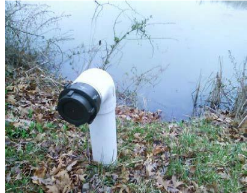
Siphon-based (Non-Pressurized) Dry Hydrant Image Source: en.wikipedia.org
