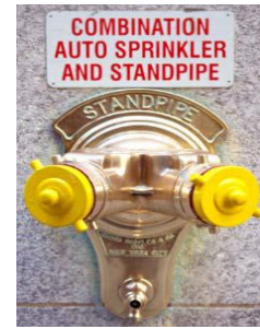
Standpipe Quick-Connect Hose Connection
