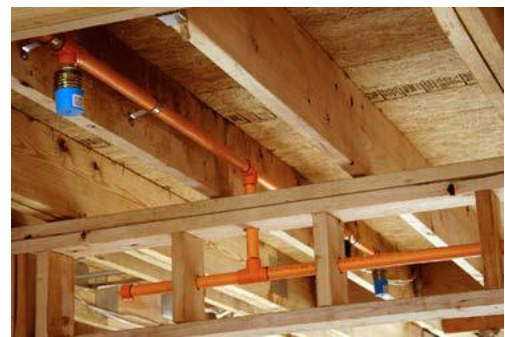
Stand-alone Residential Fire Protection System Image Source: aaspink.com
