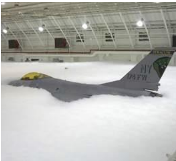
Aircraft Hangar filled with Foaming Agent from a Deluge System
