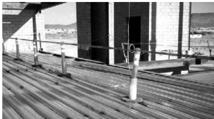
Controlled decking zone
