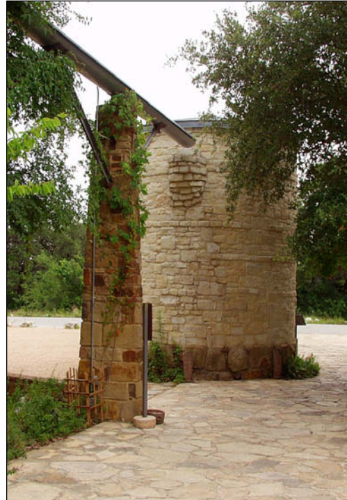
The entry cistern at the Lady Bird Johnson Wildflower Research Center is reminiscent of the stone-and-mortar cisterns used by Hill Country settlers. Water from a 1,200-square-foot roof area is conveyed to the entry cistern via an aqueduct.
