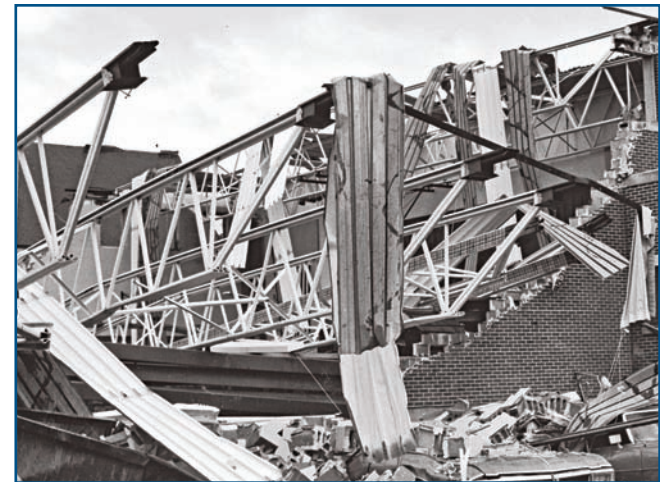
Figure 3-14 Collapsed St. Augustine Elementary School Gymnasium building.
