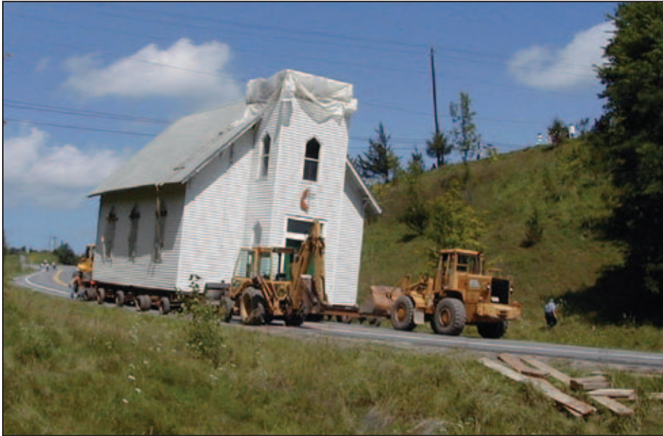
Figure 6-16. Relocation of an existing building to another location
