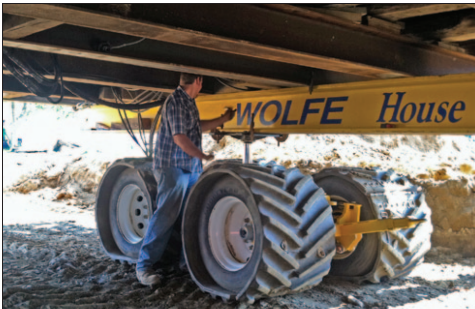
Figure 5R-11. Trailer wheel sets are placed beneath the lifting beams (photo courtesy of Wolfe House Movers)
