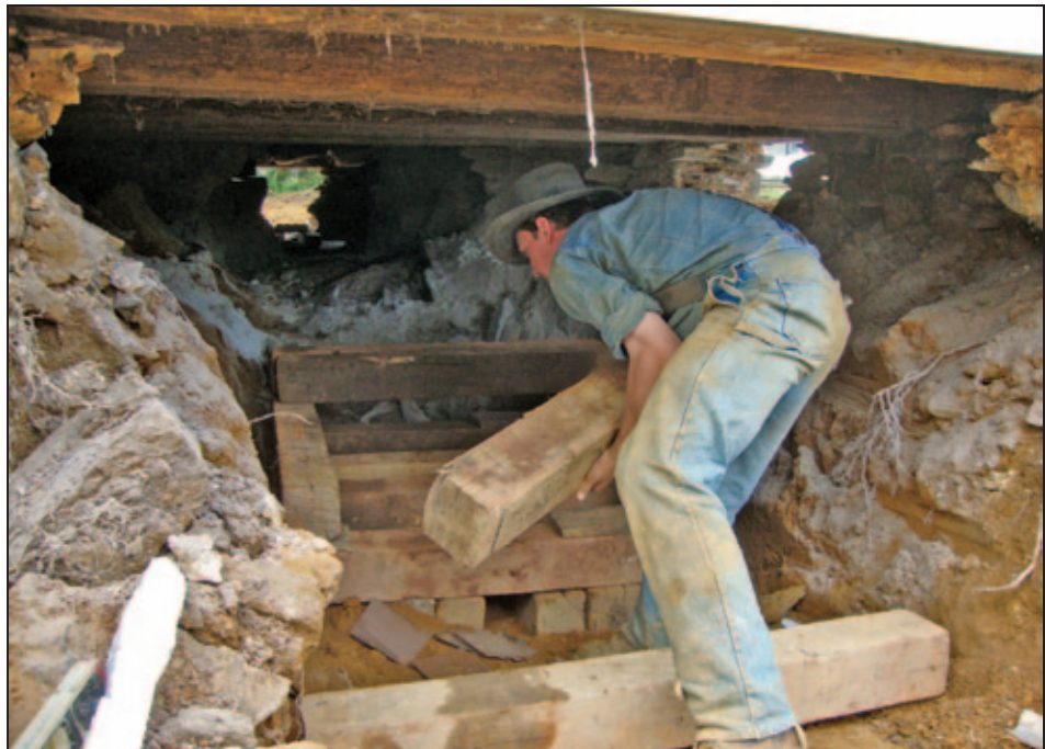
Figure 5R-5. Pathways for lifting beams (photo courtesy of Wolfe House Movers)
