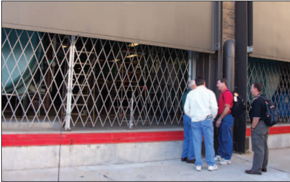
Figure 5D-39. Flood shields that can be raised and lowered to protect a hospital mechanical room from floodwaters
