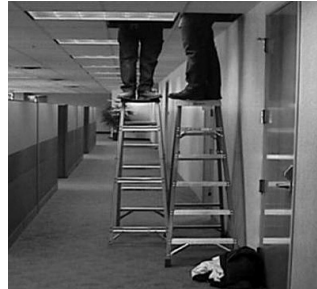
Top or top step of stepladder must not be used as a step.
