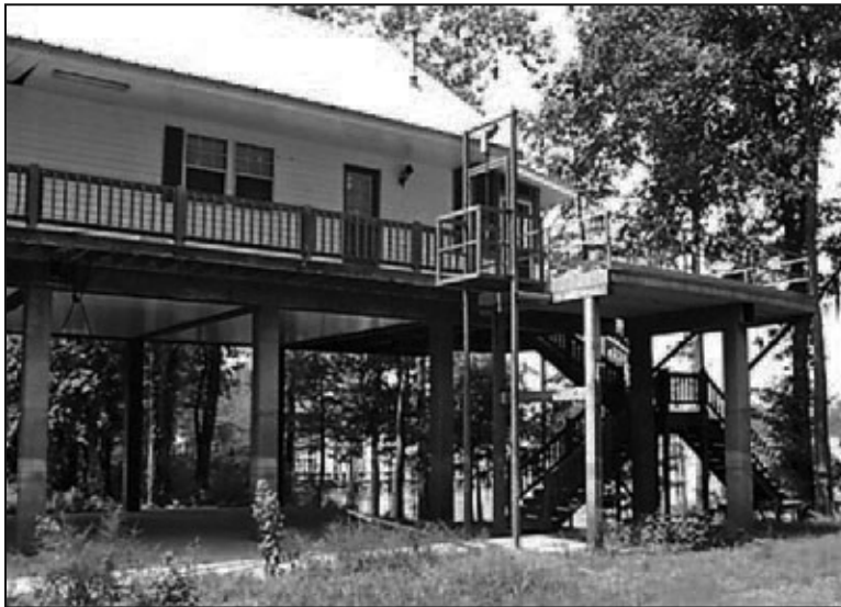
Figure 6-28. House elevated on timber piles
