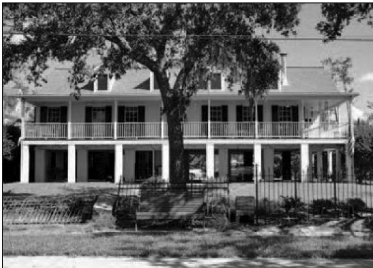
Figure 6-29. Elevation on timber piles
