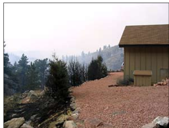
Figure 4. A noncombustible ground cover in Zone 1 helped this home survive a wildfire (Anchor Point Group, Boulder, CO).
