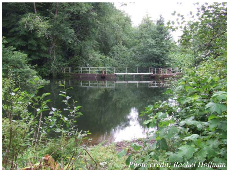
Figure 10. Coal Creek dam prior to removal
