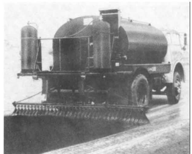
Figure 4-51. Distributor applying asphalt.
