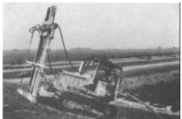
Figure 4-23. Lime slurry pressure injection (LSPI) rig treating a failed highway slope.
