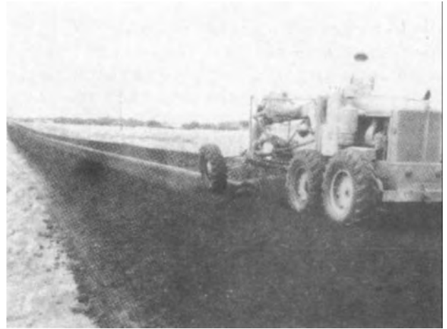
Figure 4-50. Mixing with motor grader.
