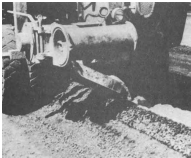
Figure 4-9. Windrow-type mechanical spreader placing cement on windrow.
