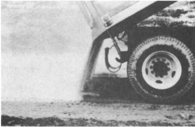
Figure 4-28. Spreading of granular quicklime.
