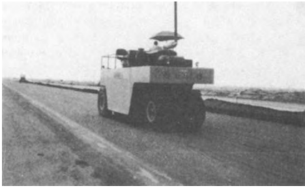
Figure 4-42. Pneumatic roller completes compaction of LCF base.
