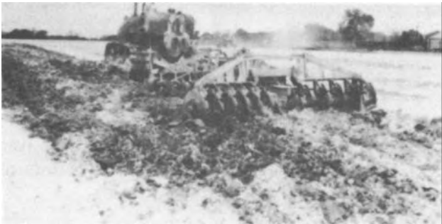
Figure 4-36. Mixing with a disc harrow.
