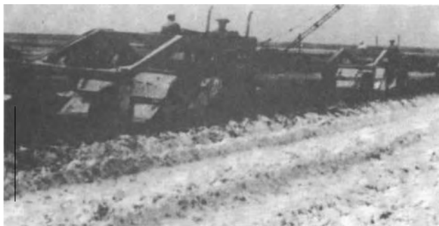
Figure 4-38. Train of rotary mixers.
