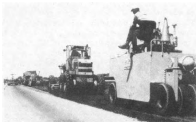
Figure 4-52. Spreading and compacting train.
