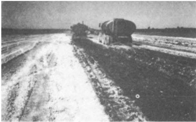
Figure 4-35. Watering of lime-treated clay on airport project.
