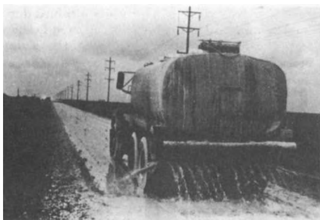
Figure 4-31. Spreading of lime slurry.
