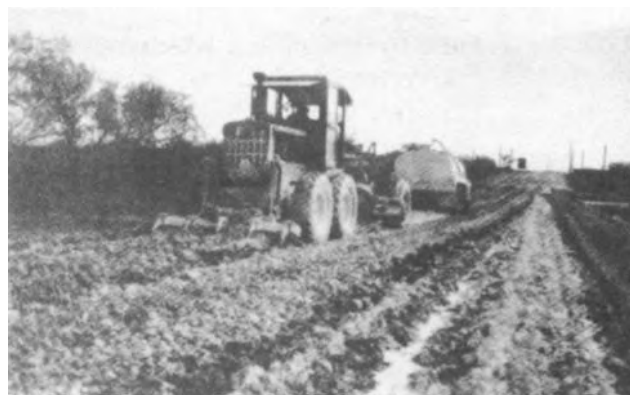
Figure 4-33. Grader-scarifier cutting slurry into stone base.
