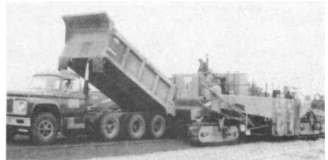
Figure 4-56. Spreading cold mix with full-width cutter-trimmer modified for paving.
