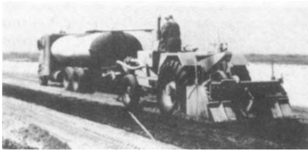
Figure 4-48. Single-shaft rotary mixer with asphalt supply tank.
