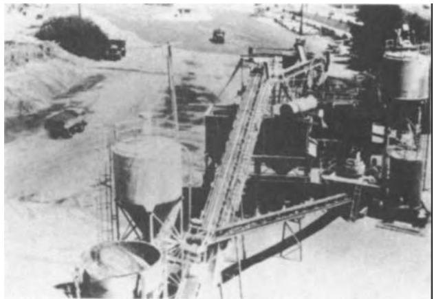
Figure 4-22. Enclosed soil holds lime for adding to marginal crushed stone base material.
