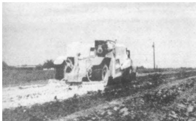
Figure 4-32. Recirculation pump on top of a 6,000-gallon wagon agitates the slurry.
