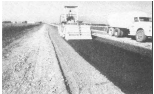
Figure 4-39. Rotary mixer on primary road project.
