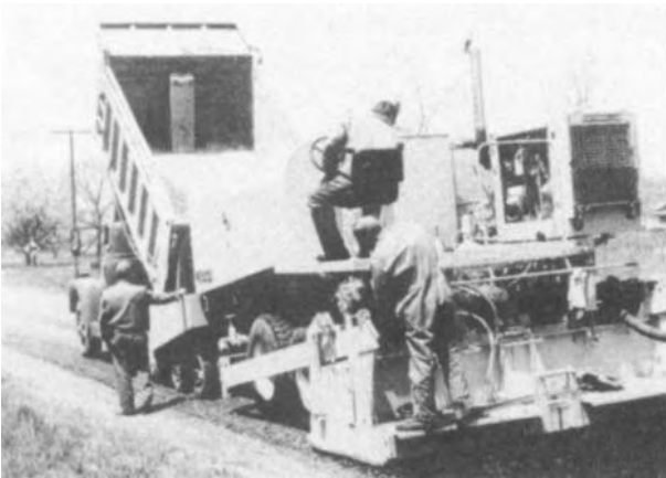
Figure 4-45. Hopper-type pugmill travel plant.
