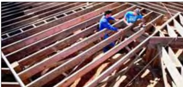
Pressure-treated Southern Pine 2x10 floor joists.
