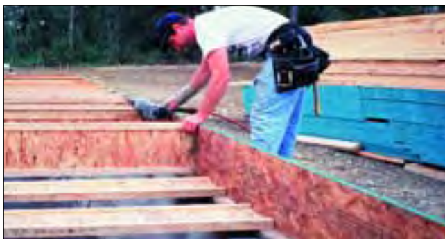
Rim board attaches to prefabricated I-joists.
