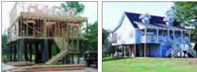
Storm surge protection in hurricane-prone coastal areas requires an elevated floor system. Wood piles are also an option for this application.
