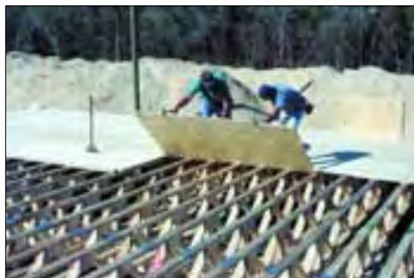
Workers install subfloor sheathing over floor trusses of a 5,000 sq. ft. assembly building. See case study D, page 43.
