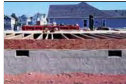
Vent openings in a stem wall foundation provide cross ventilation.
