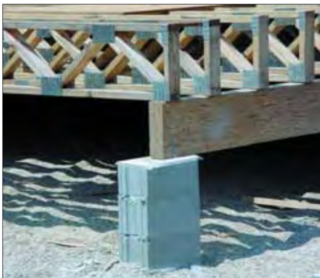
Structural composite lumber beam supports floor trusses.
