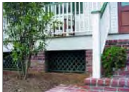
The ground beneath an open pier-and-beam foundation should be graded to provide drainage away from the structure.
