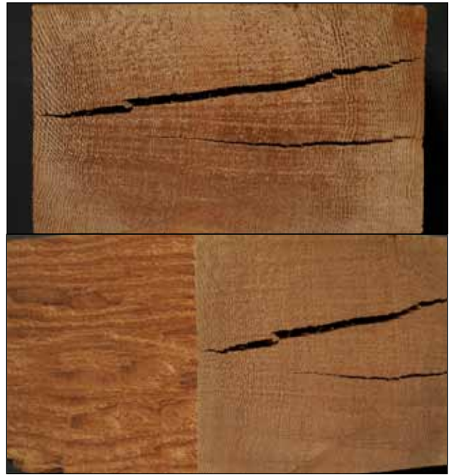
Figure 13-11. Red cedar timber end shows honey-comb (top). Surface of the timber shows no honey-comb (bottom).
