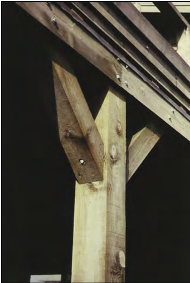
Figure 13-9 Knee bracing in a wood-pile foundation.
