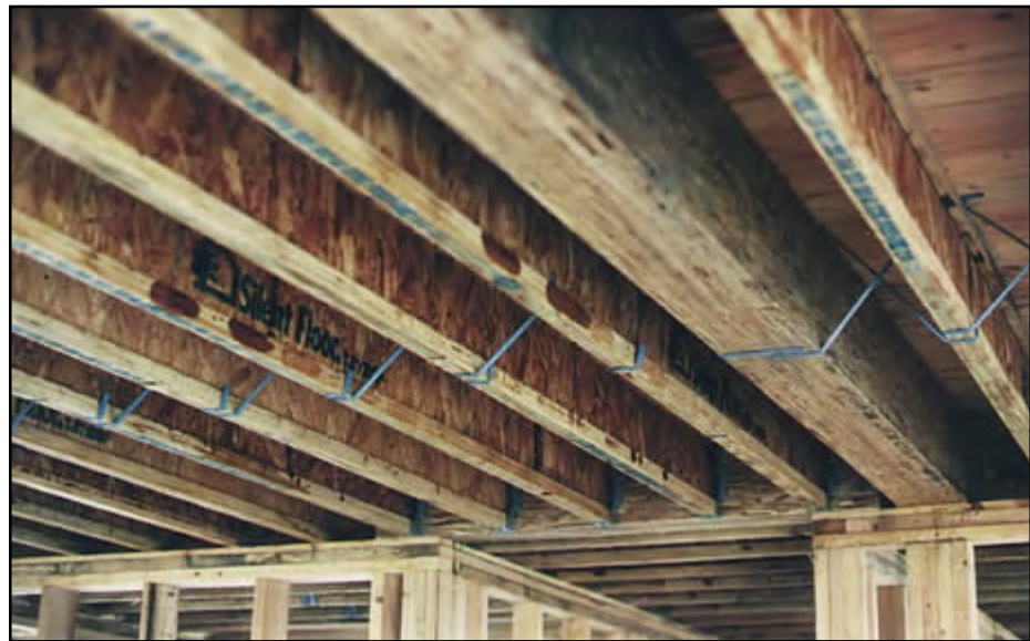
Figure 13-24 Plywood web I-beams used as floor joists with metal brace used to keep the bottoms of the joists from twisting. Also note glue-laminated beam.
