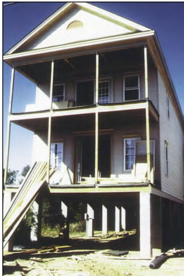
Figure 13-10 Open masonry foundation.
