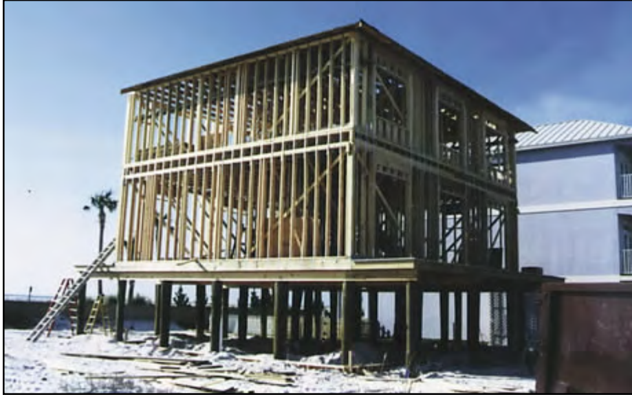
Figure 13-7 Typical wood-pile foundation.
