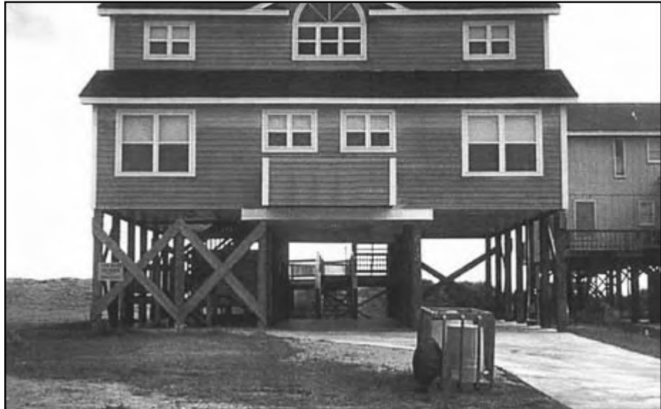
Figure 13-8 Diagonal wood bracing in a wood-pile foundation.
